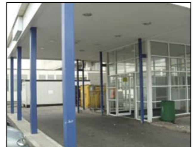
THE entrance to the new-look maternity unit nears completion.
