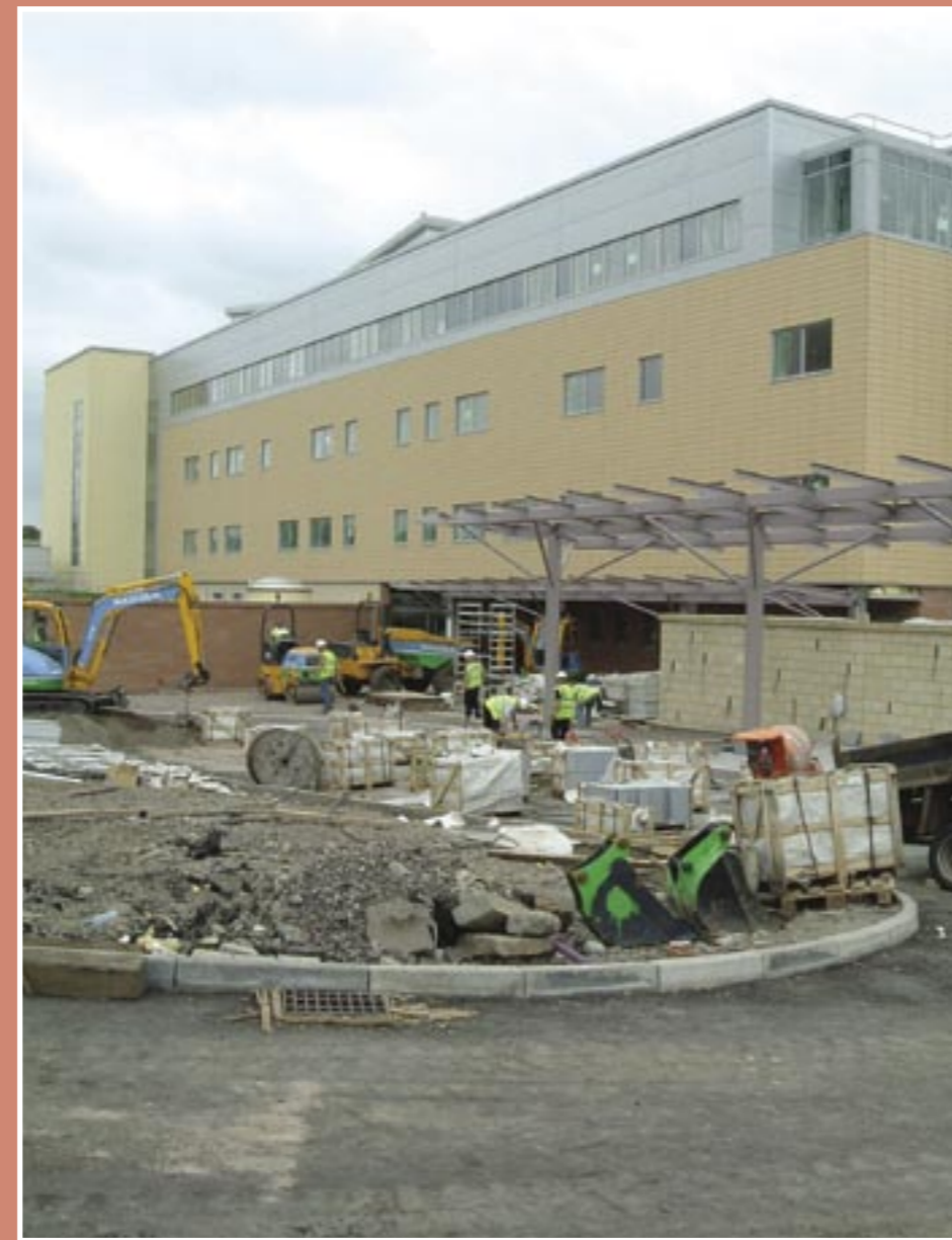
WORK is still underway at the main entrance to the Beatson.
